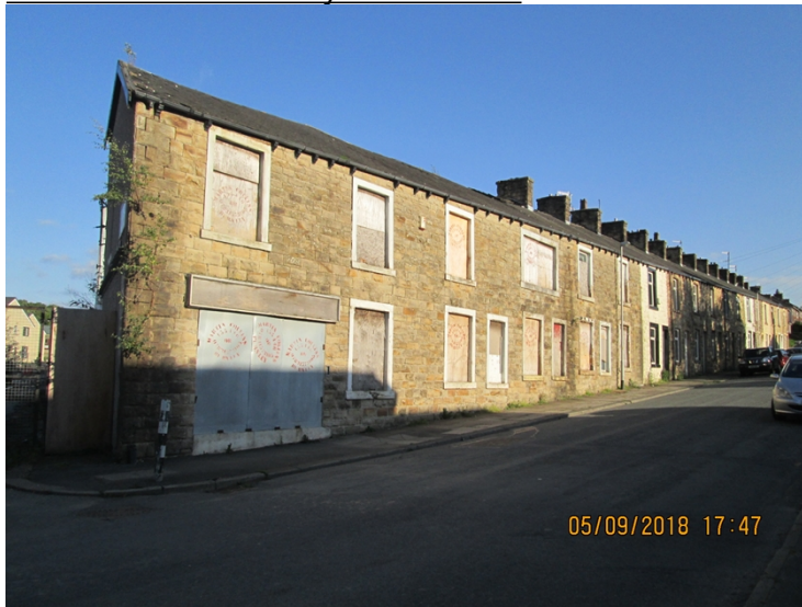
Former offices on Wytham Street
