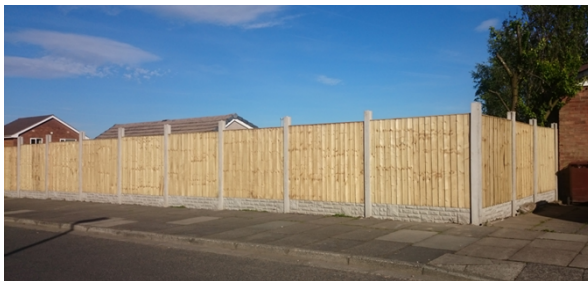
View of existing fence from Parkwood Ave.
