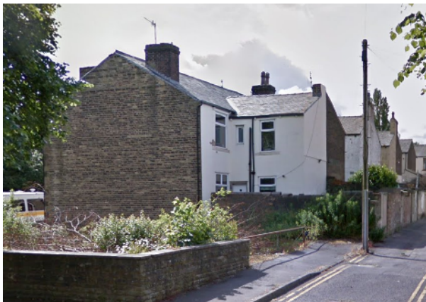
No. 3 Fairview Road showing the position of windows
