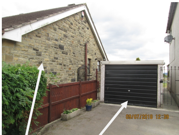
no.15 and existing garage to no.13
